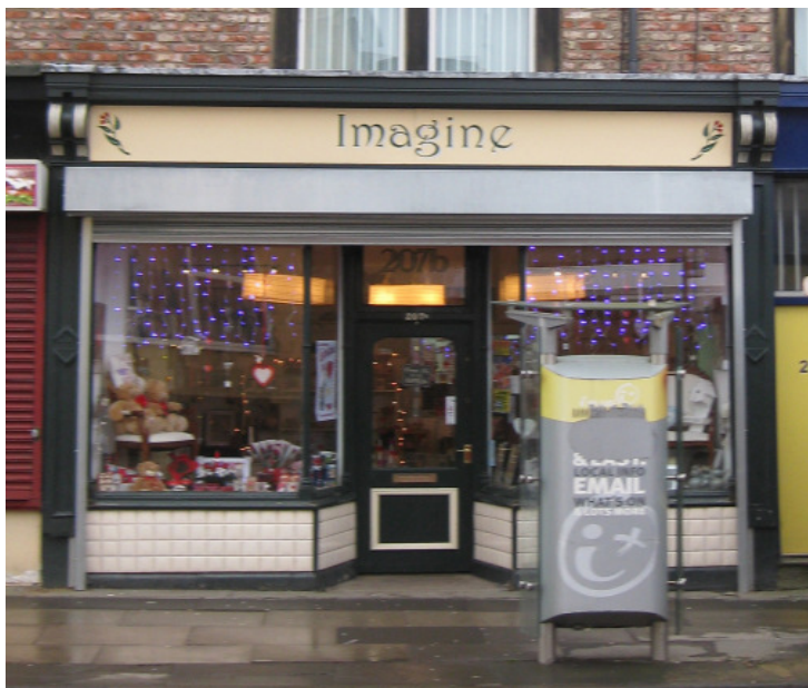
“Inappropriate use of tiles at stallriser”
