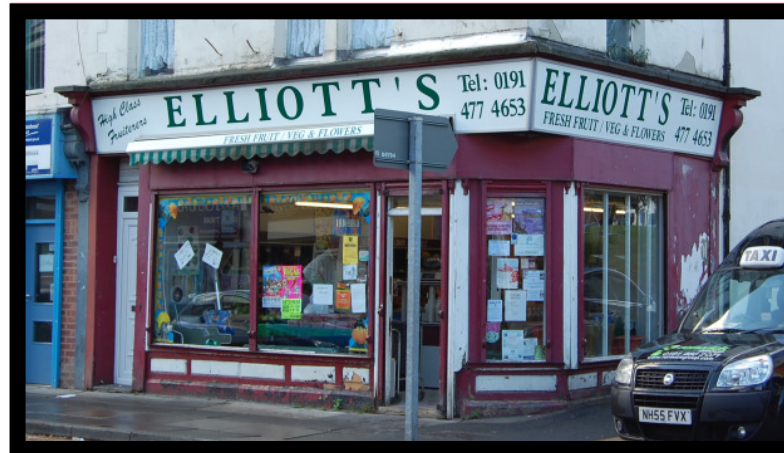
A SIMPLE TRADITIONAL TIMBER SHOPFRONT, ALTERED BUT WITH MOST COMPONENTS IN PLACE
